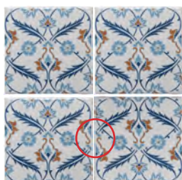
This is incorrect as the patterns on the sides do not line up, because the tile bottom right is upside down
